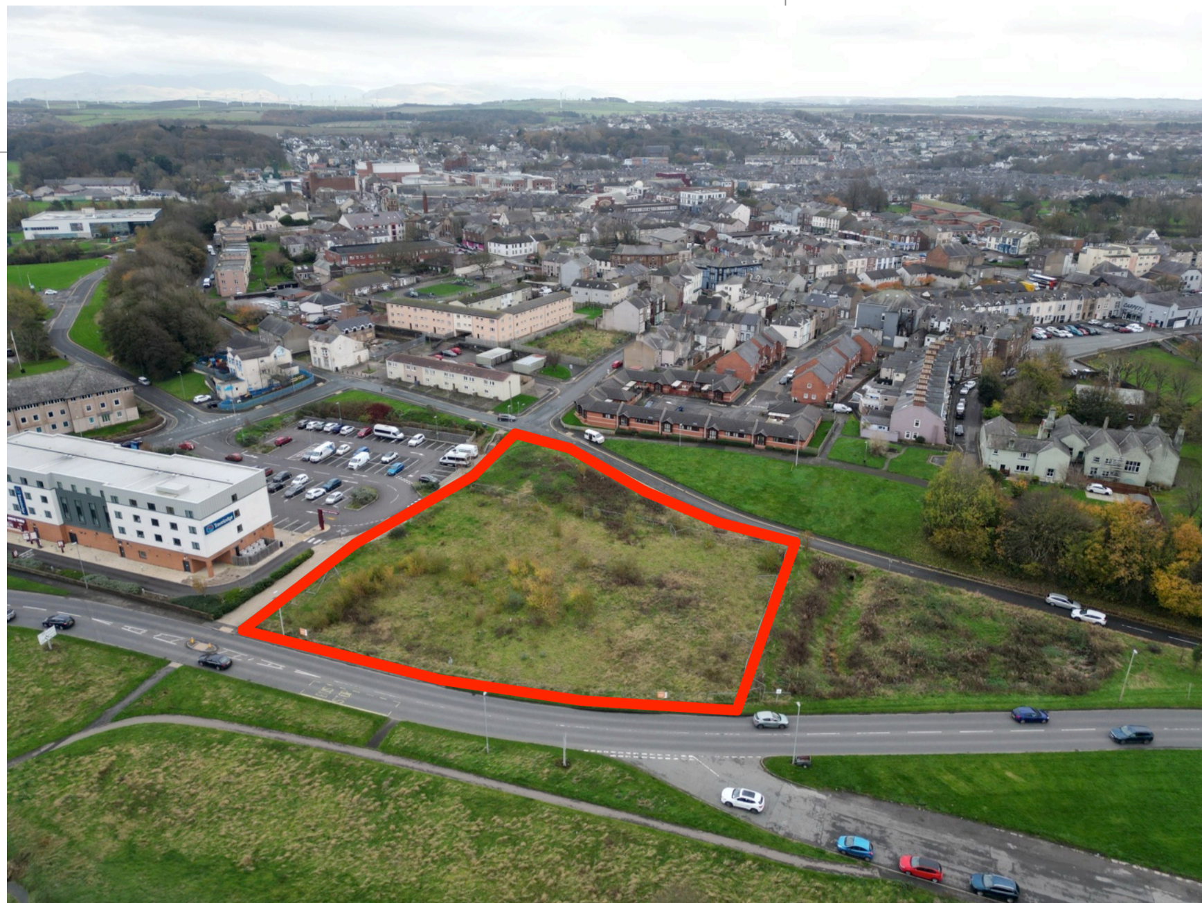
AERIAL VIEW OF SITE
