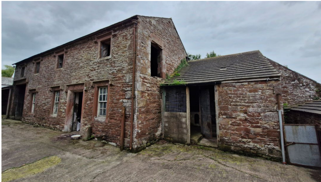
PHOTO 02 VIEW ON RIGHT HAND GABLE AND EXTENSION
