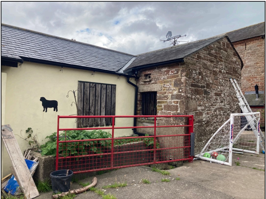
Figure 7: Byre and barn tie-in area - both roofs are modern and have no suitable access for bats and the walls do not provide crevices - wall tops also do not present gaps or access to suitable voids / crevices.
