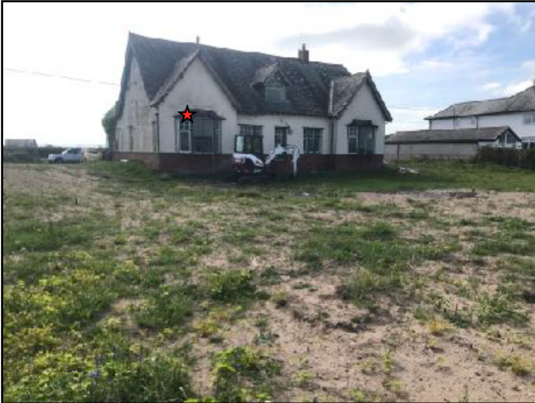
Figure 9: Showing the western elevation of Sandy Lodge with active starling nest (1 of 2) identified via red star.
