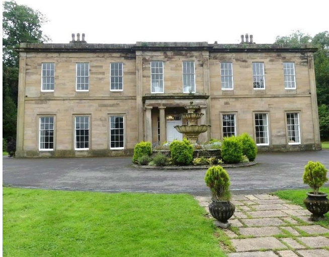
The front elevation of The Fitz
