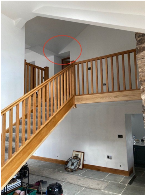
Illustration 6 –View of Entrance hall and staircase Steelwork spring point set out by door head height (highlighted in the red circle)
