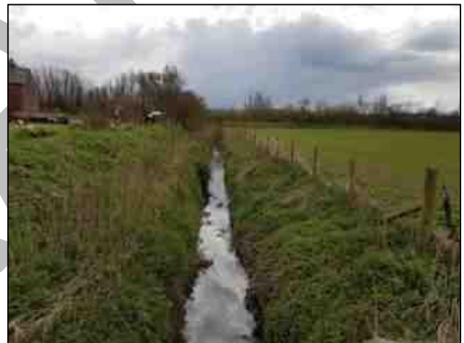
Photograph 17: Spittal Farm Drainage Channel
