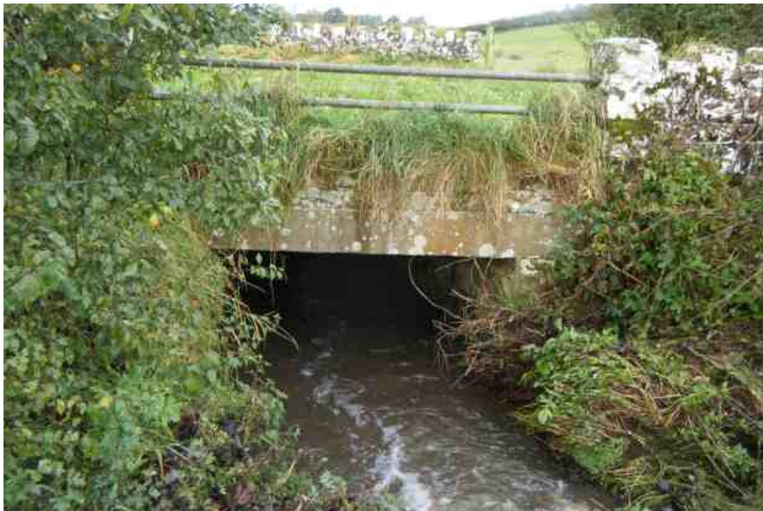
Photograph from site visit (JBA – October 2012)
