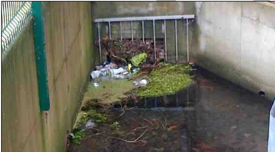
Photograph 12: Trash Screen on the Tributary Next to Lidl
