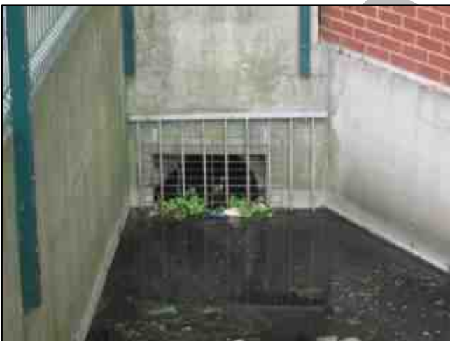
Photograph 14: Lidl Trash Screen
