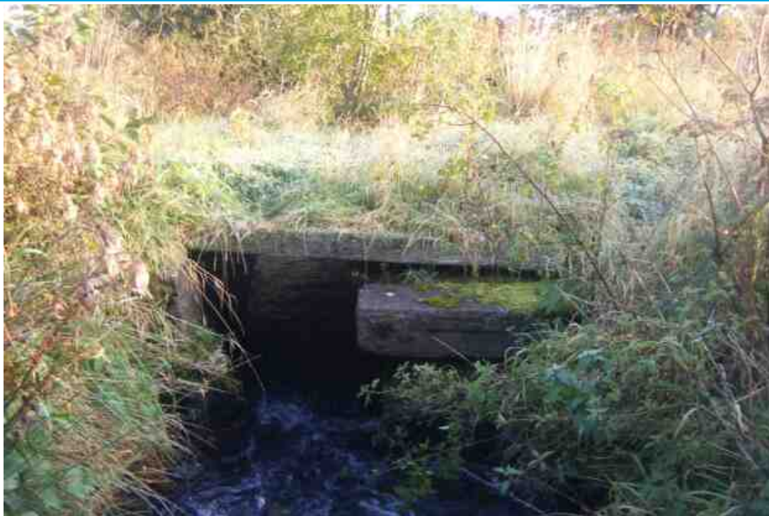
Photograph from site visit (JBA - October 2012)
