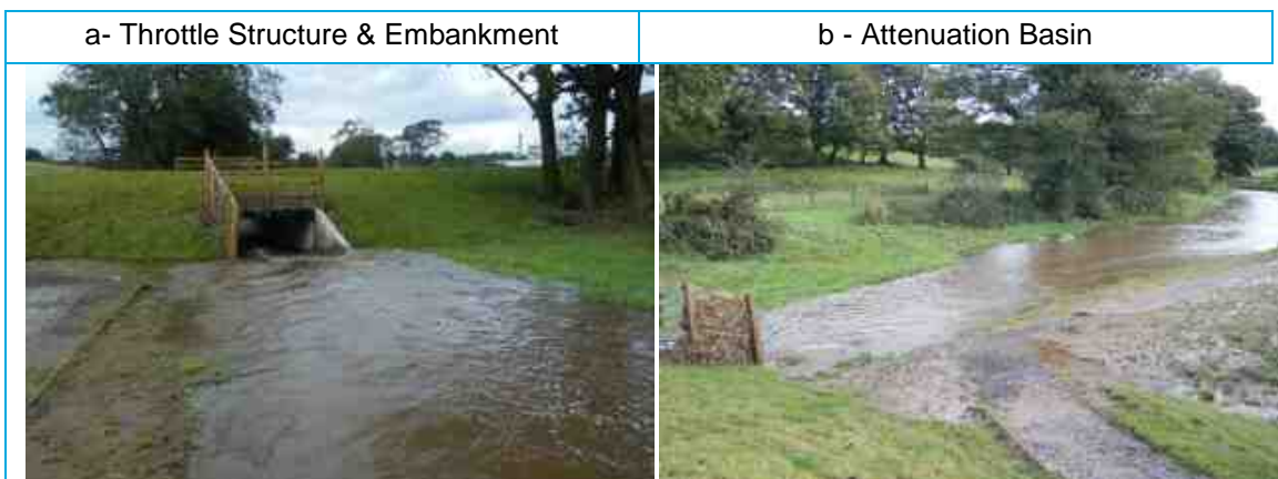
Figure 3-4: Wiza Beck Flood Retention Basin: structures
