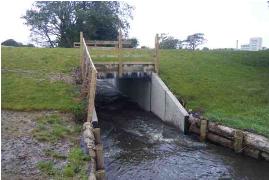
Photograph from site visit (JBA - October 2012) – Throttle Structure
