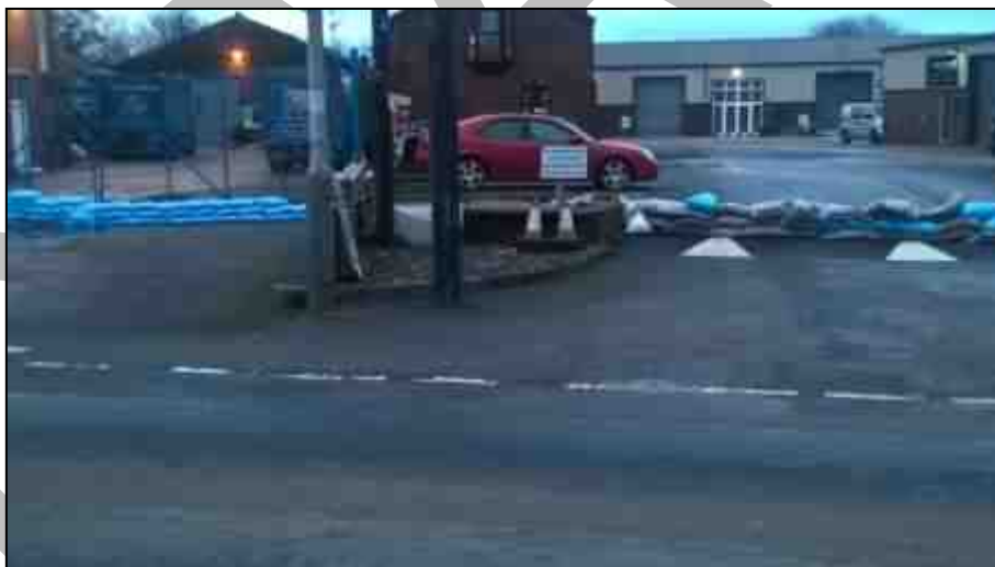
Photograph 6: Temporary Sandbags and bags of salt on Station Road (7 th Dec 2015)
