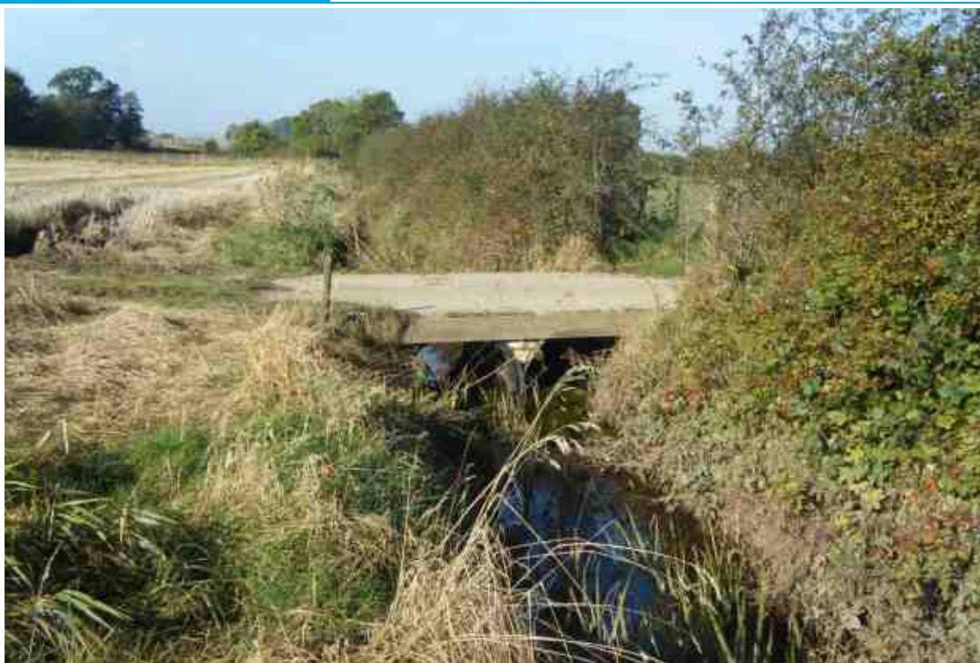
Photograph from site visit (JBA - October 2012)
