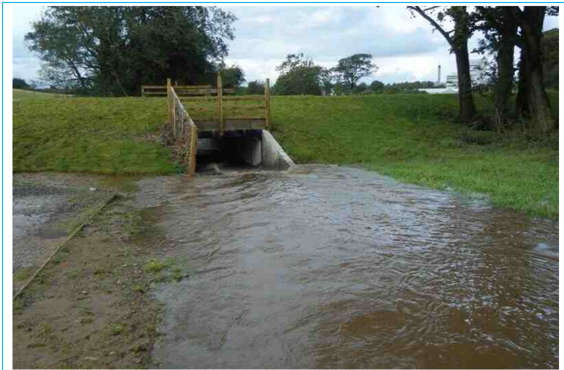
Figure 1-2: Wiza Beck throttle structure
