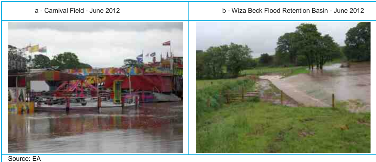
Figure 2-4: Photographs of flooding in June 2012
