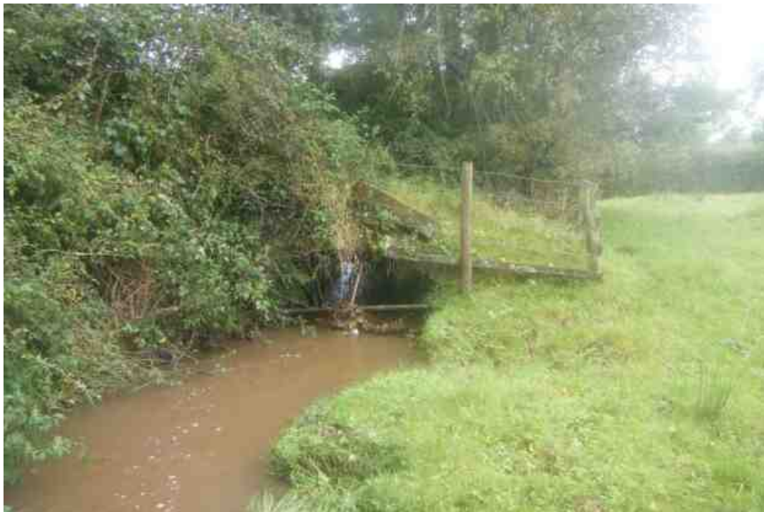
Photograph from site visit (JBA – October 2012)
