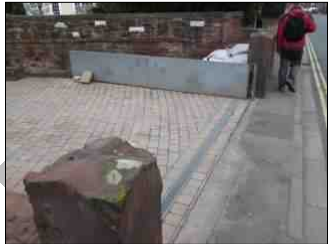
Photograph 8: Flood Gates on Station Road
