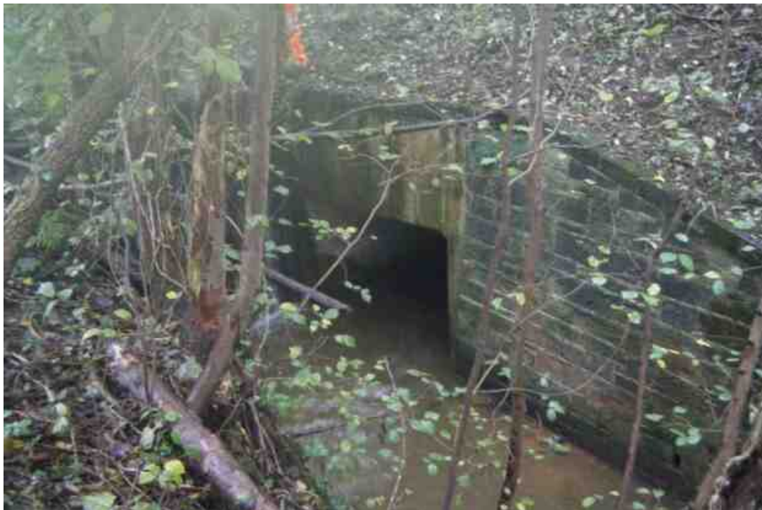
Photograph from site visit (JBA - October 2012)
