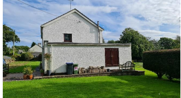
Photograph 2: North aspect of garage
