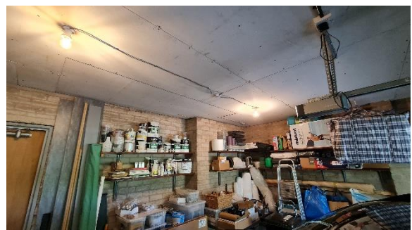
Photograph 2: Internal photograph showing brick walls and lined ceiling
