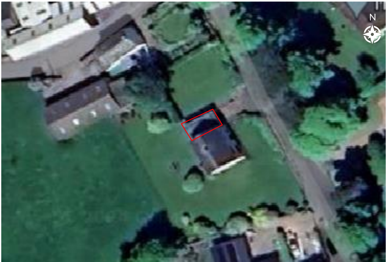
Figure 1: Brandle How building, with location of works highlighted in red.
